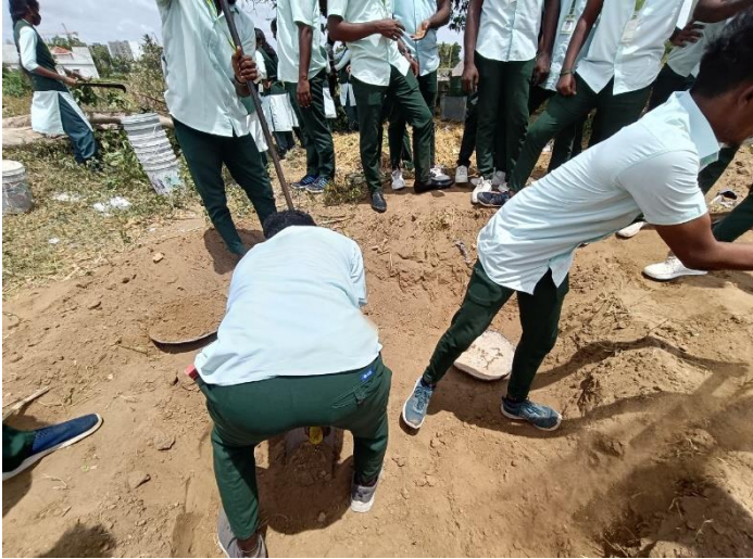
Digging of Compost Pit
