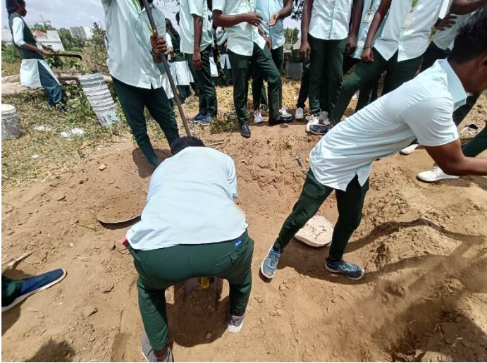
Digging of Compost Pit
